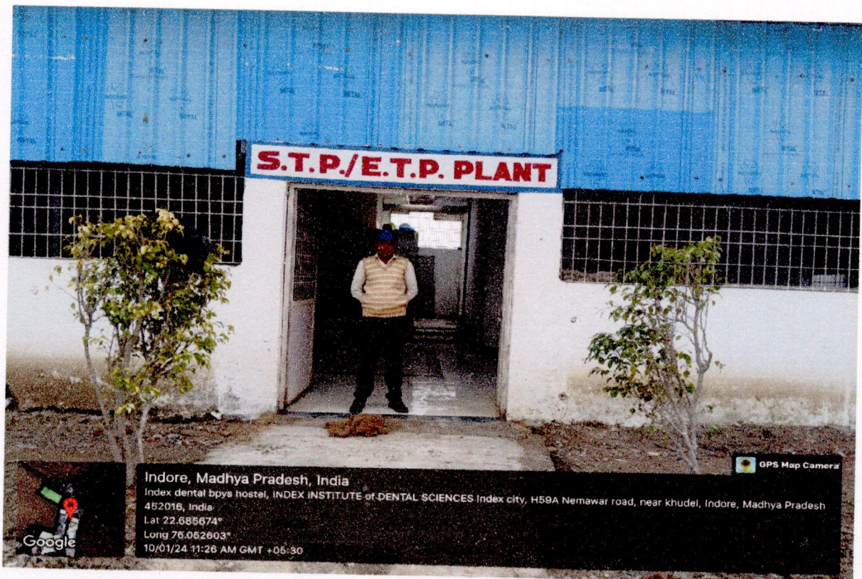
Photo: Sewage Treatment Plant (500 KLD)
